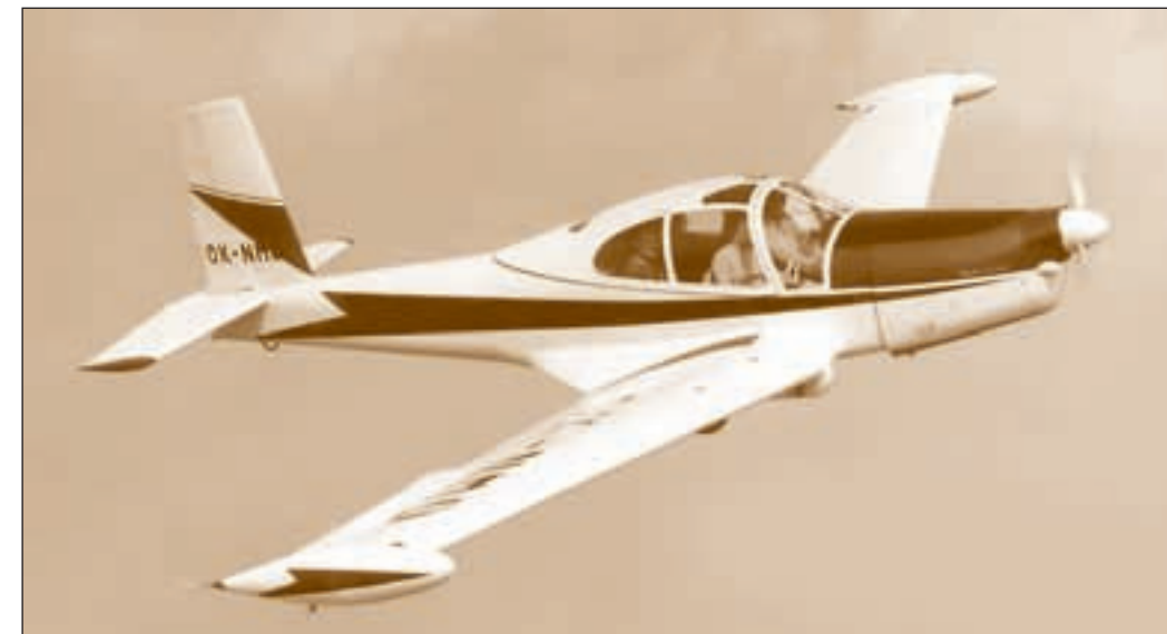
Four seater L-40 Meta Sokol with additional tanks
