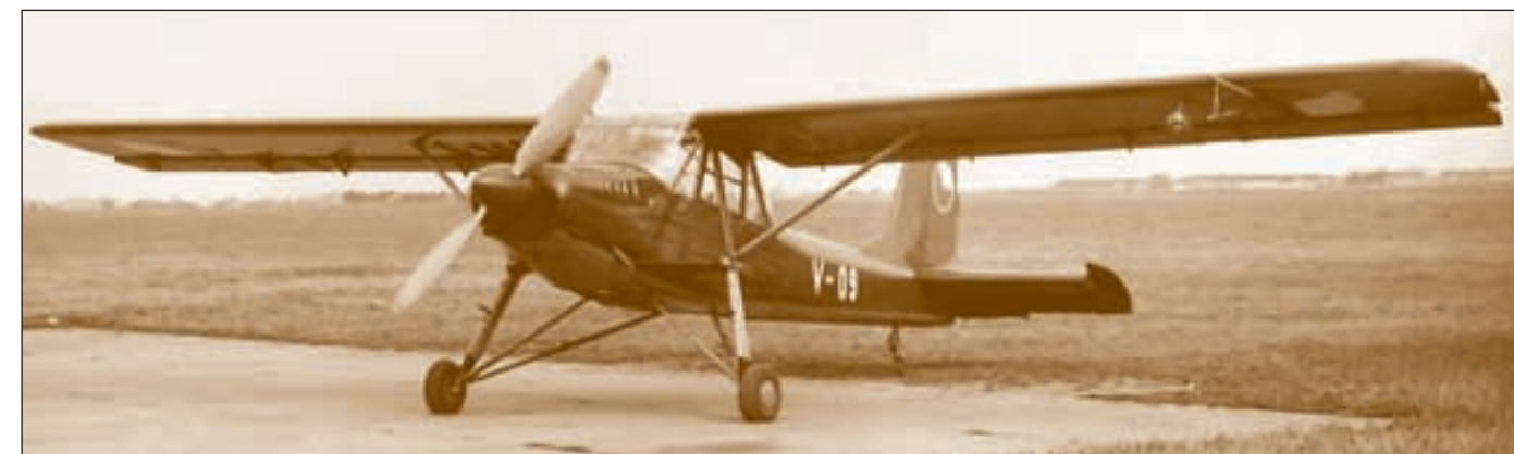
Upgraded from L-60 Brigádýr, L-160 featured one beam wing, largely metallic skin structure and simple struts. No batch production
